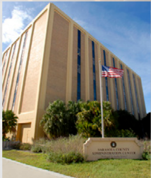
County Administration Building
